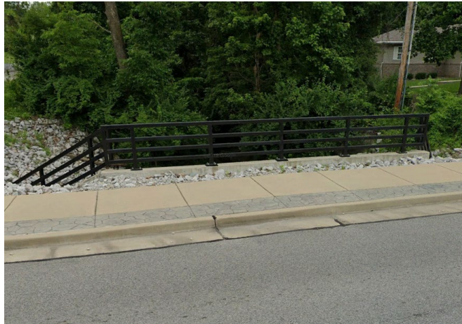
Bridge Rail Barrier
