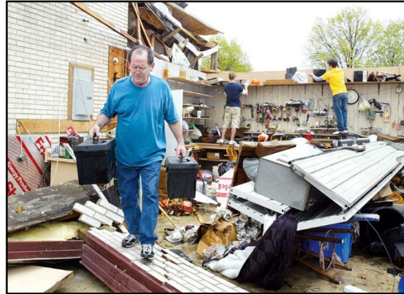
Structure damage sustained along Maryville Road in Granite City during the April 22, 2011 EF2 tornado.
