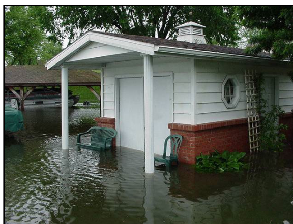
Flash flooding on May 25, 2009 damaged over 100 homes in Holiday Shores.
