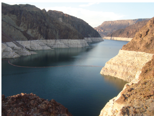
Figure 6.1. Decreasing water levels in Lake Mead impede hydroelectric power generation (Mjiponso (talk)/Wikimedia Commons (CC BY-SA 3.0))
