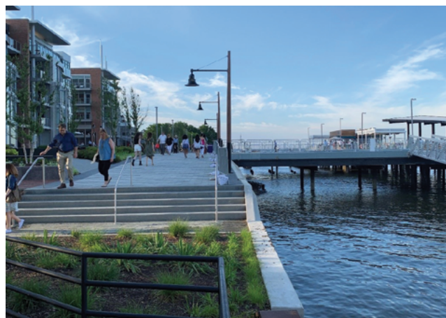
Figure 9.10. Robinson Landing promenade adaptation project (Robert Kerns)
