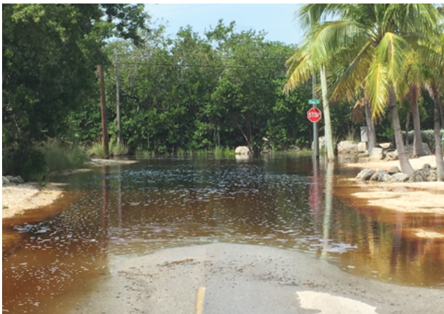
Figure 9.12. October king tide road flooding in Key Largo, Florida (Erin Deady)
