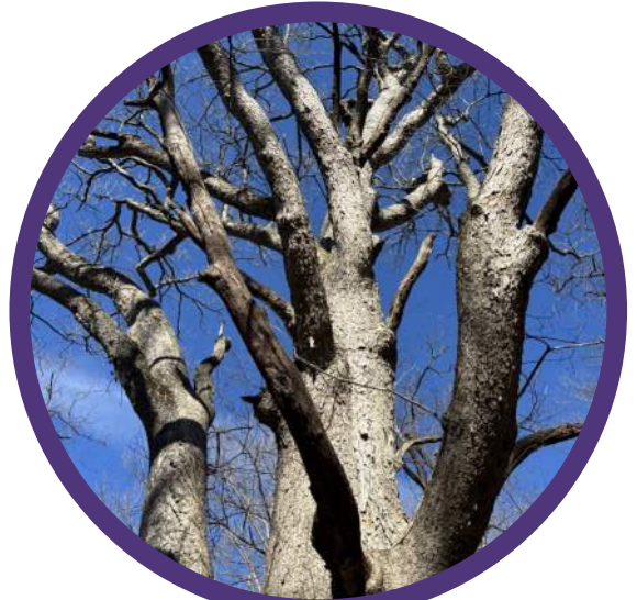
Dead/Dying Trees - Falling Limb Hazards
