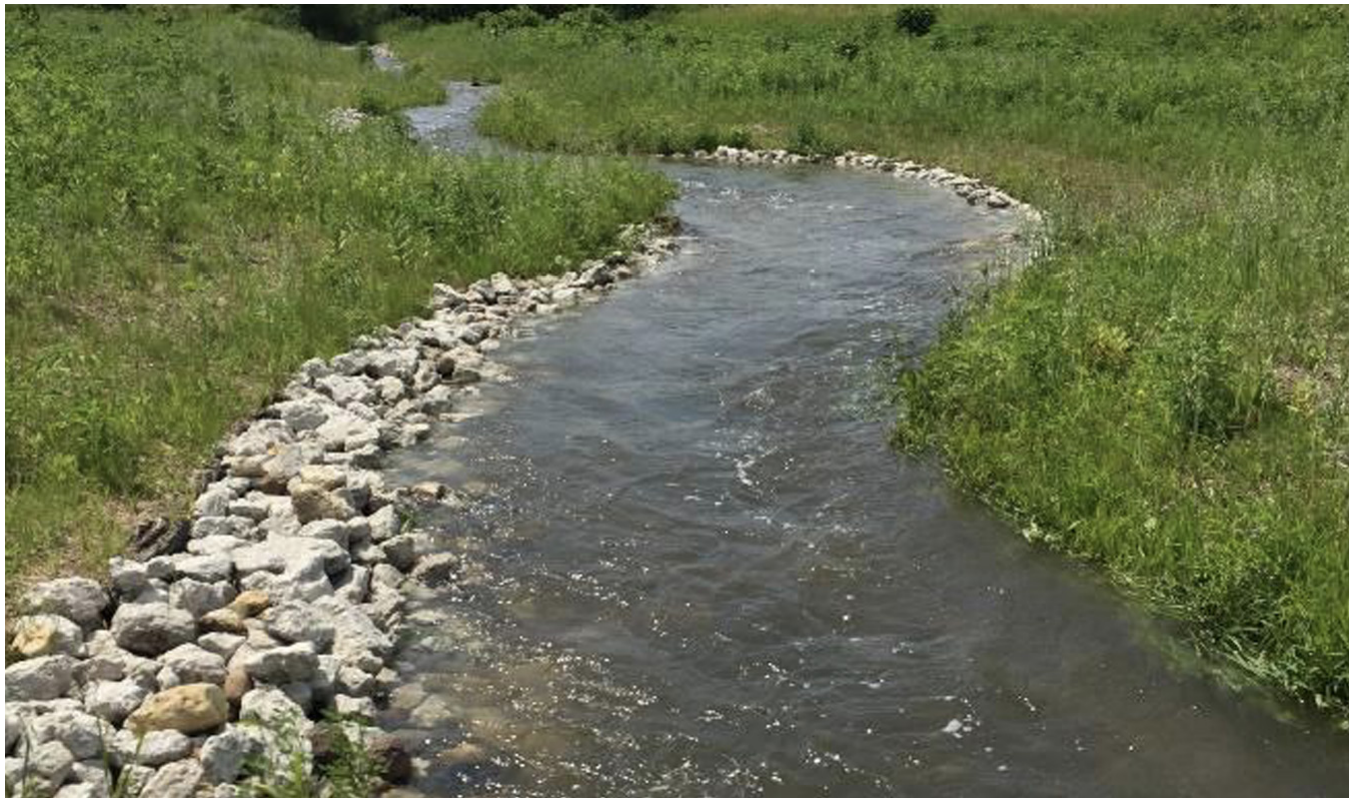
Below PC: IEPA - FAA 3191608 – The Woods Creek Stream-bank Stabilization and Restoration project stabilized eroding streambanks on Woods Creek by widening the channel and installing a floodplain shelf, a riparian buffer of native vegetation, stone toe protection, and rock riffle grade control structures.
