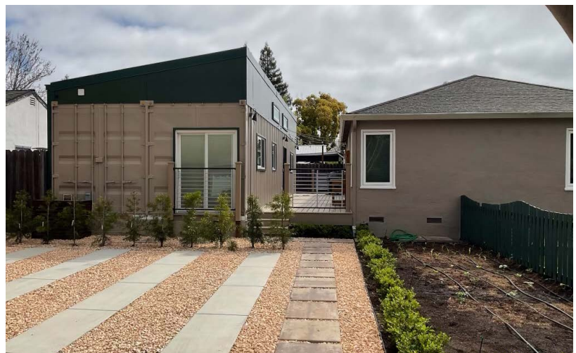
■ An accessory dwelling unit constructed from a shipping container (Credit: Kubed Living)
