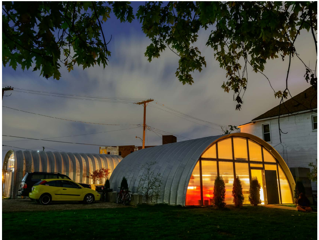
Quonset homes in the True North Quonset village in Detroit (Credit: SteelMaster Buildings/Flickr )
