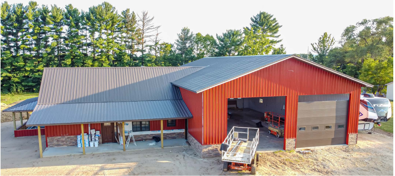
A barndominium under construction in Trempealeau County, Wisconsin (Credit: Wikideas1/Wikimedia Commons )
