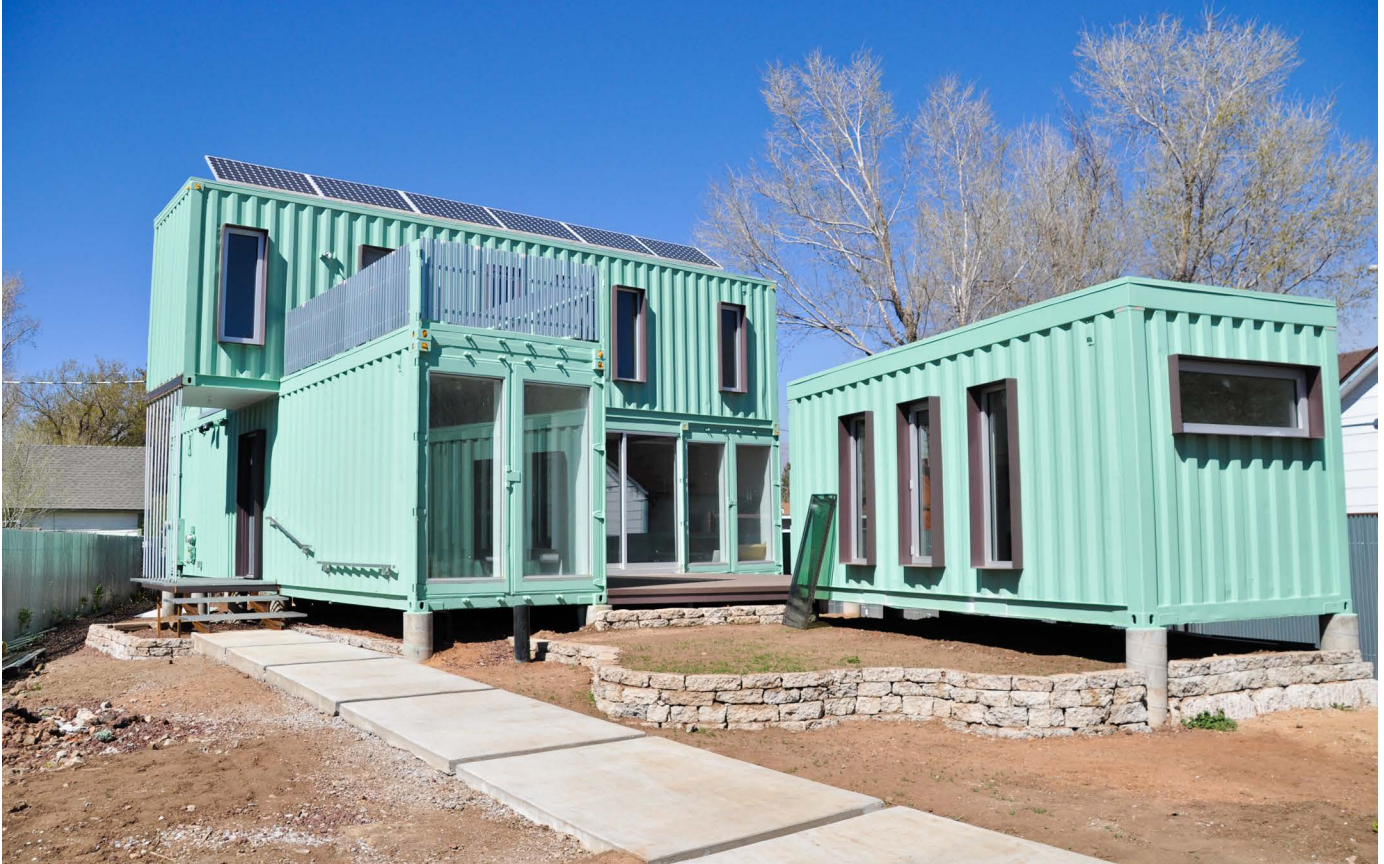
■ A shipping-container home in Flagstaff, Arizona (Credit: Tom Check/Flickr )
