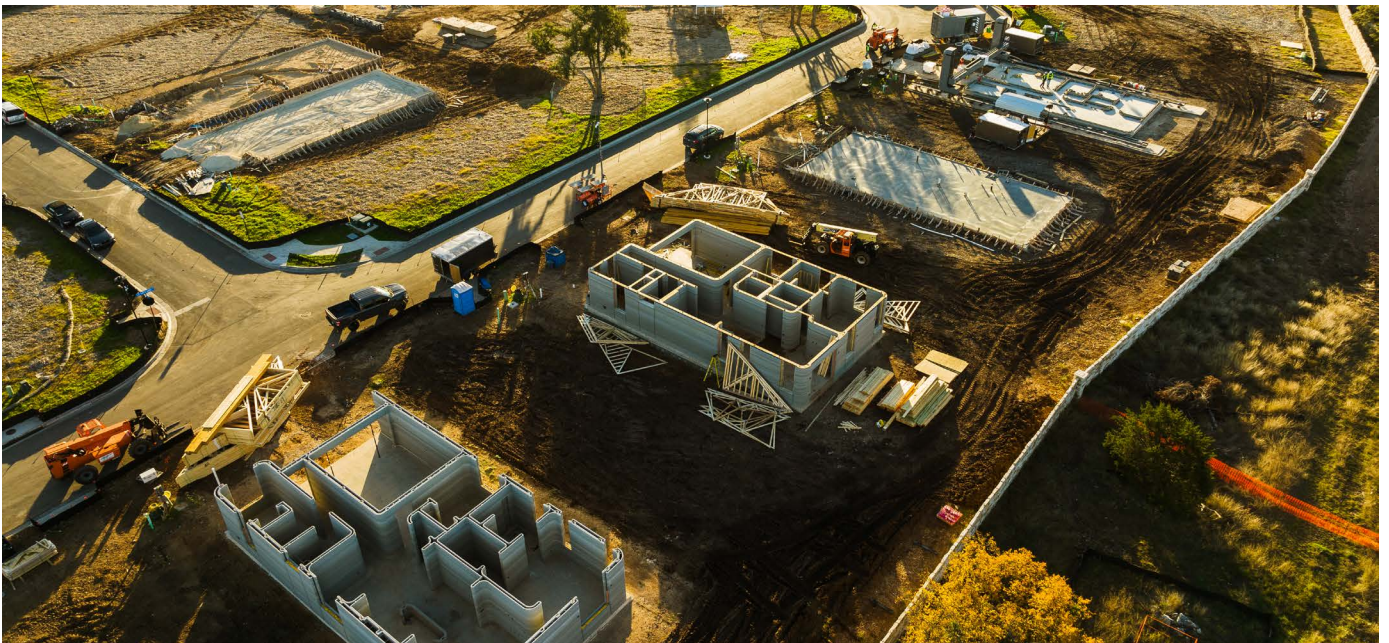
3D-printed homes under construction near Austin, Texas (Credit: Roschetzky/stockPhoto/iStock/Getty Images Plus)
